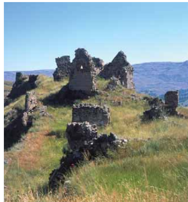
325. Tmkaberd Castle, Javakhk, from the north-east 326-328. A partial view of the castle ramparts; cut-in-rock steps descending towards the river Kur, and remnants of castle buildings
