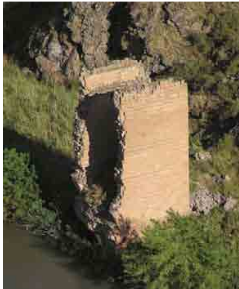
673-675. Bridge piers over the river Akhurian in Ani, Kars Region
