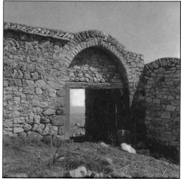
Khalash. Gate of the Bek's house
