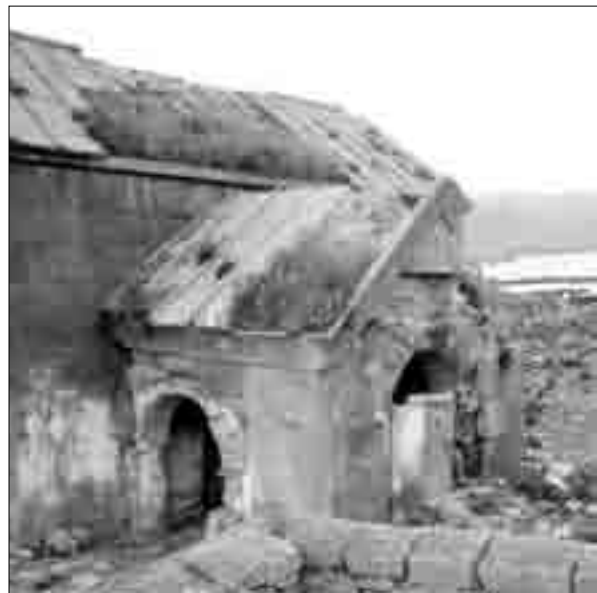
ABUL. Sourb Harutiun (Holy Resurrection) Church seen from the south-west and north-west; its entrance-hall from the south-west
