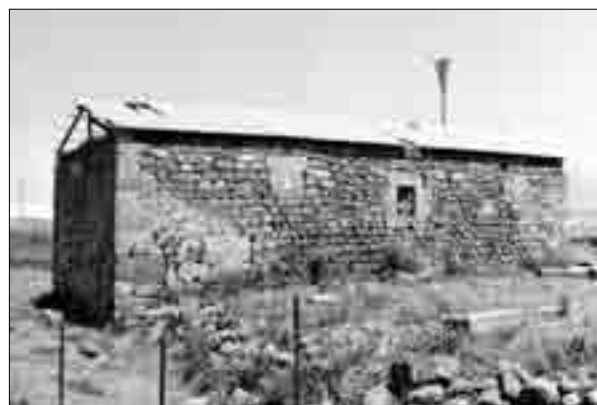
NAMZARA. Soub Lusavorich (Holy Enlightener) Church as seen from the east, south-east, north-east and south
