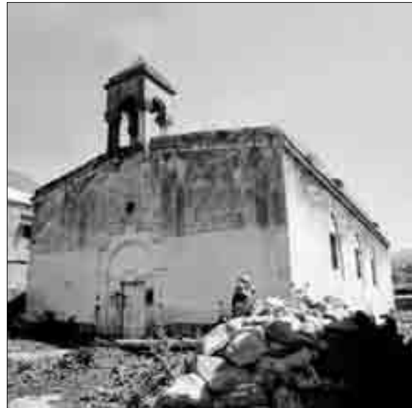
BALKHO. St. Sahak Partev (Sourb Harutiun) Church as seen from the south-west
