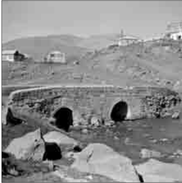
GANDZA. A bridge over the river Parvana
