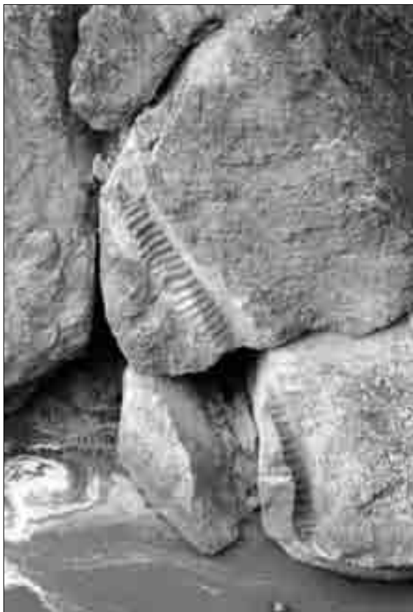
TMOK (TMKABERD). The cut-in-rock underground passage leading to the riverside
