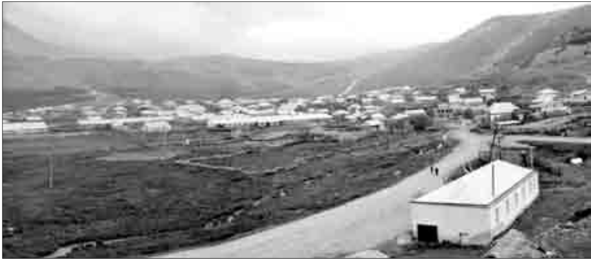
ABUL. The village seen from the south-west
