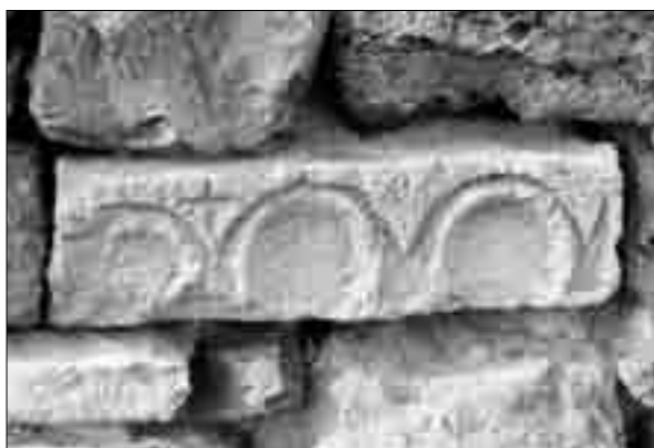
KORKH. The inscription (1890) commemorating the renovation of St. Stepanos Church; a chapel, and a cornice fragment from an early medieval church set in the wall of the chapel
