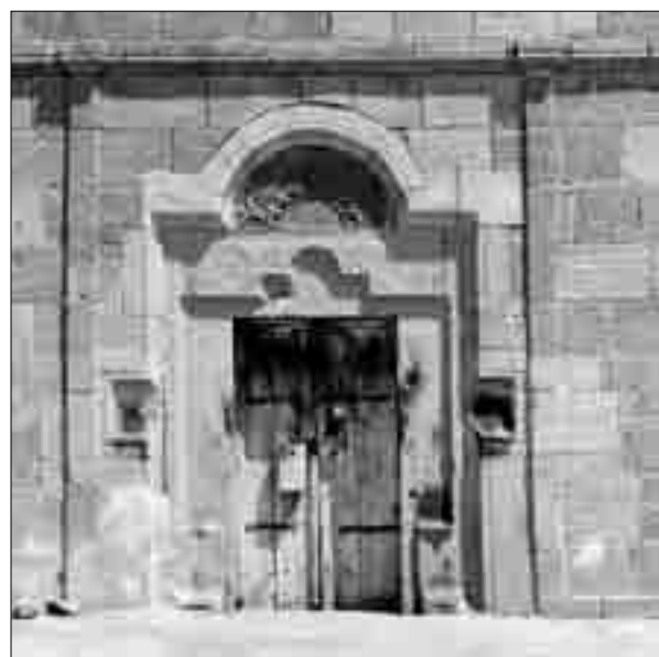
POKR KHANCHALI. St. Hakob Church as seen from the south-west, and its entrance opening from its western facade
