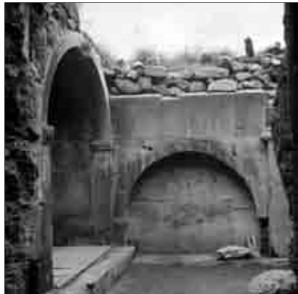
BAVRA. The older church of the village as seen from the north-east and west; a partial view of the section adjoining the bema of the hall church which stands in the south of the sanctuary
