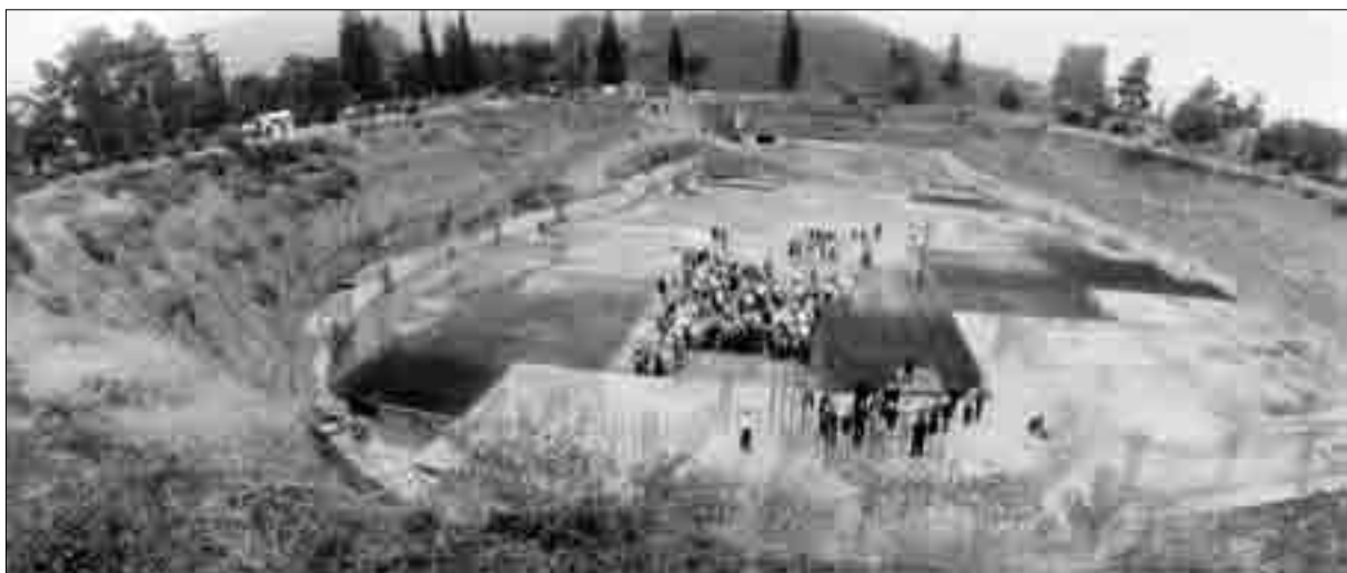
The foundations of the future church (photos by S. Darchinian)
