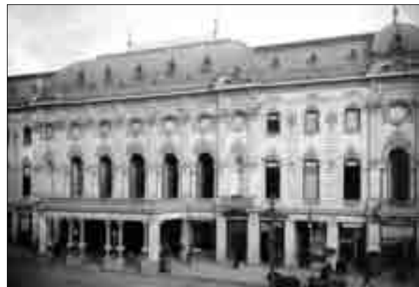
The edifice of the Artistic Society (nowadays: Rustaveli Theatre) built by Yesayi Pitoyan
