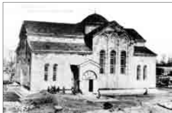
GANDZAK (GYANJA). St. Grigor Lusavorich Church before the construction of its dome
