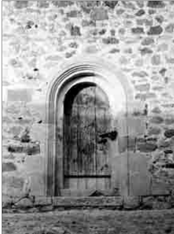
NUKZAR. St. Gevorg Church seen from the south-west and west
