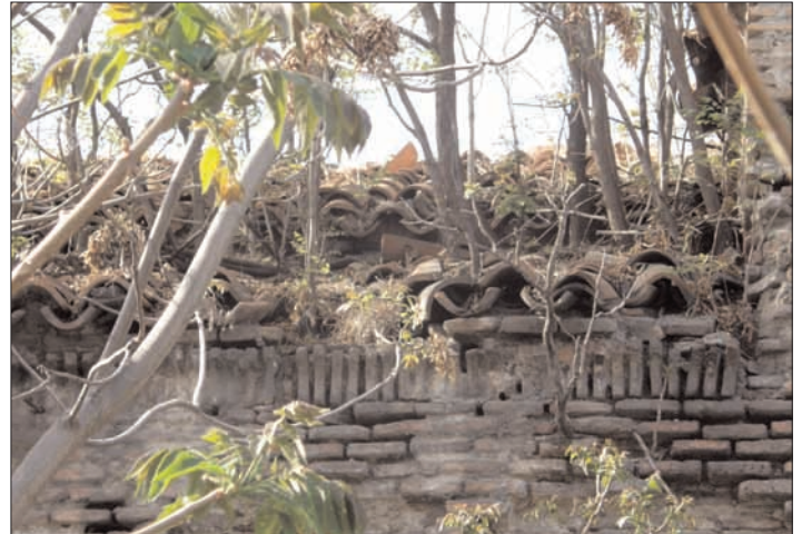
The tiled roof of the church, which was seriously damaged by the conflagration of 2002, easily fell prey to vegetation in the subsequent years (photos by N. Akopov, 2011 & S. Karapetian, 2007)
