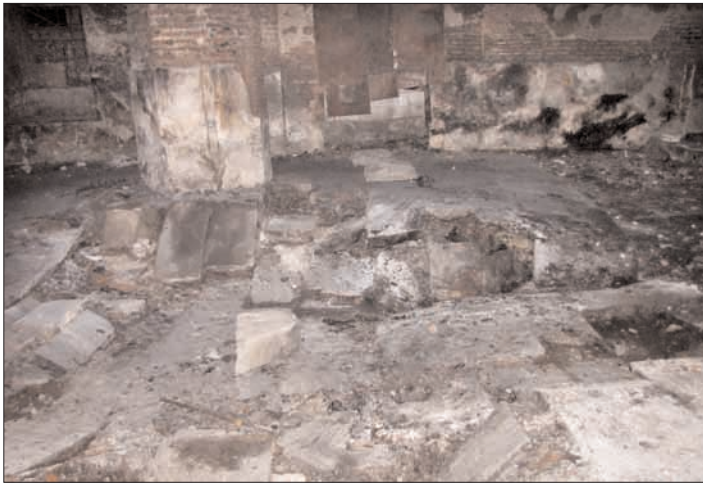
The sediments accumulated in the central part of the prayer hall and in the porch standing in front of the northern entrance: they were deposited from the water with which the fires of January 2012 were extinguished (photos by N. Akopov, 2012)
