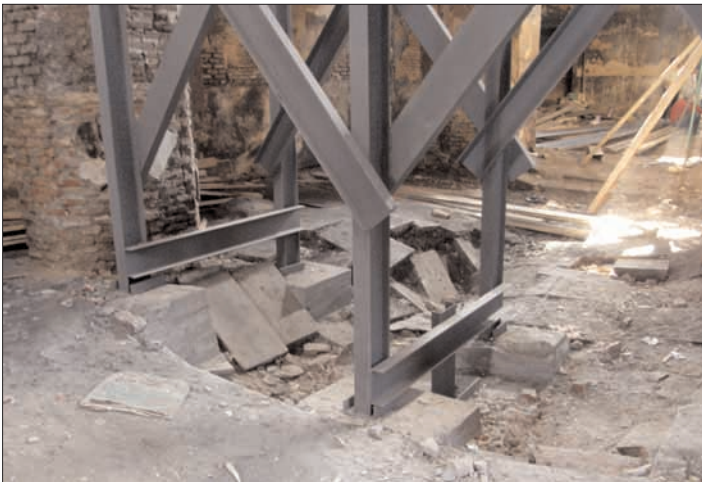
The metallic and wooden constructions placed inside the church between March and April 2012 to prevent the possible collapse of the monument (photos by A. Hakobian)
