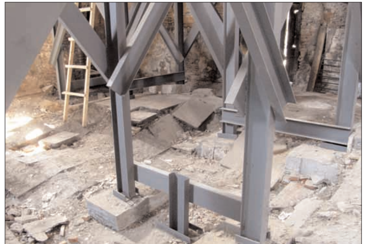
The metallic and wooden constructions placed inside the church between March and April 2012 to prevent the possible collapse of the monument (photos by A. Hakobian)
