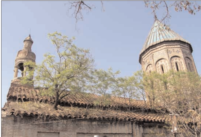
The tiled roof of the church, which was seriously damaged by the conflagration of 2002, easily fell prey to vegetation in the subsequent years (photos by N. Akopov, 2011 & S. Karapetian, 2007)
