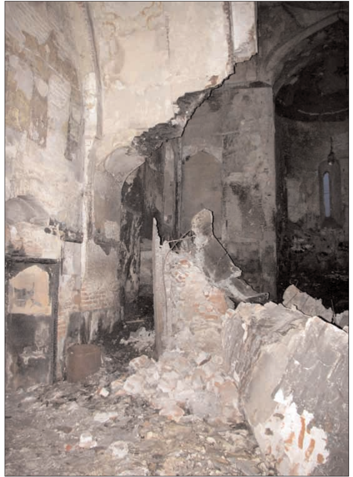
The successive fires of 3 & 7 January 2012 destroyed the north-eastern pillar of the church (they were extinguished in a manner impermissible for historical monuments—with water (photos by N. Akopov, January 2012)
