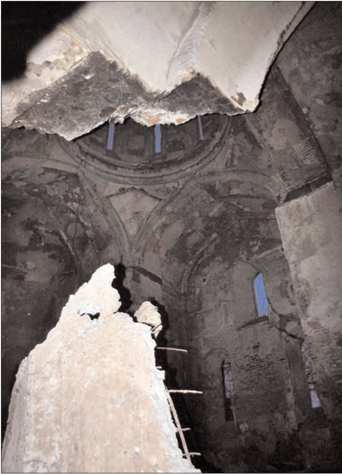
The successive fires of 3 & 7 January 2012 destroyed the north-eastern pillar of the church (they were extinguished in a manner impermissible for historical monuments—with water (photos by N. Akopov, January 2012)
