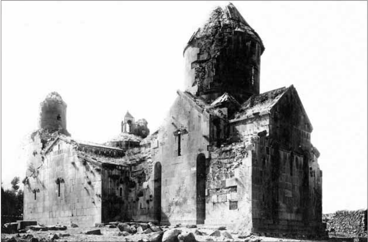
Tegher Monastery from the south-east (photo by T. Toramanian, 1924)
