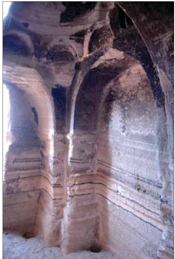
The fake dome of the south-western chapel of Tzarakar Monastery; its interior to the sanctuary (north); its north-western squinch and south-western wall pylon
