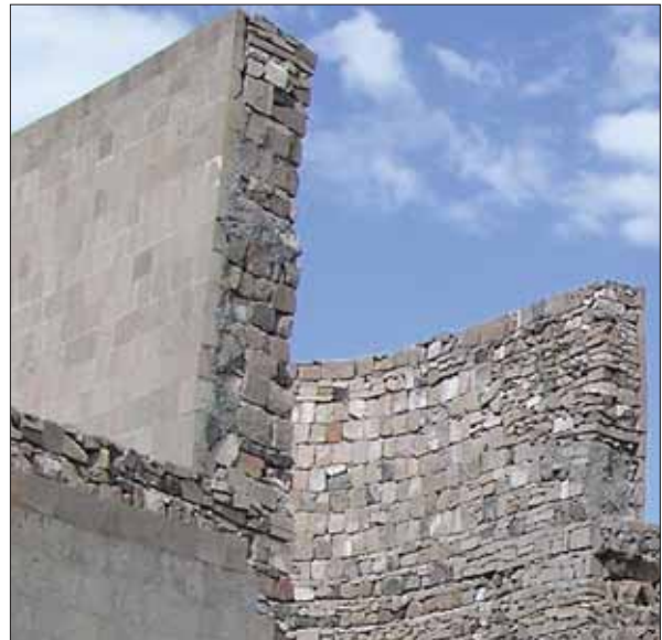
ANI. The towers adjoining the Principal Gate before and after their "restoration"; a partial view of a "restored" tower
