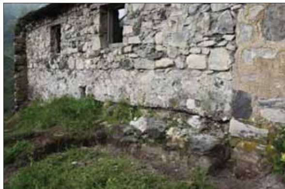
The unearthed thick retaining wall
