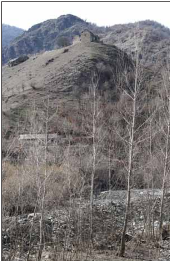
A general view of Charektar Monastery from the north-east
