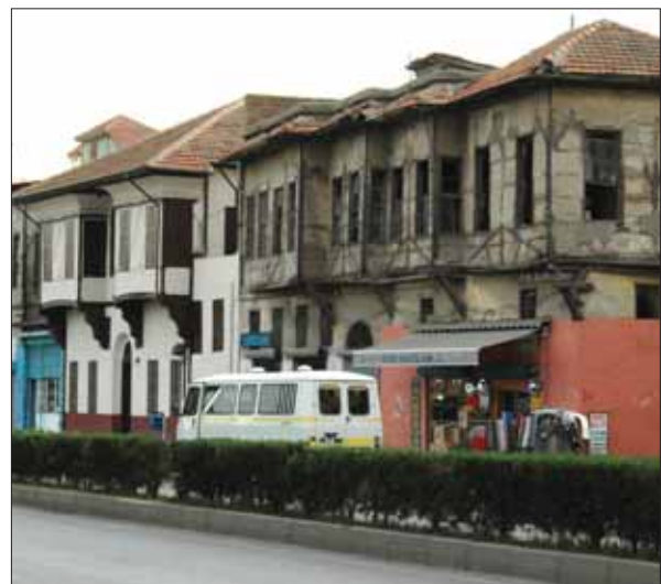
ADANA. A restored house
