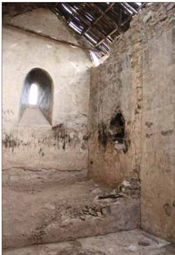
The church floor as flattened with mortar
