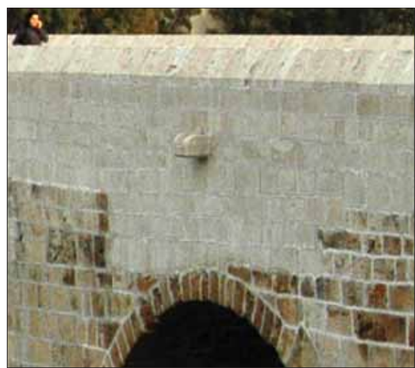
ADANA. General and partial views of a restored bridge
