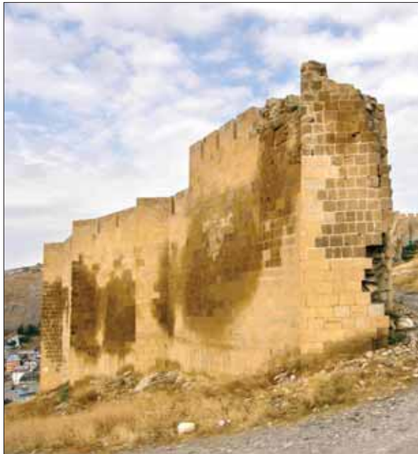
BABERD. Partial views of the “restored” castle ramparts
