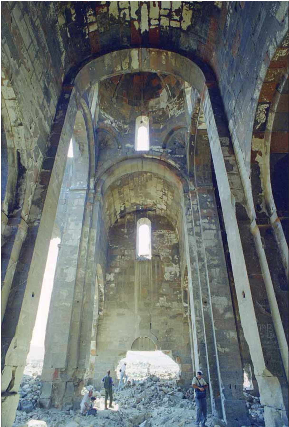
Mren. The interior of the cathedral to the west (photo 2000)
