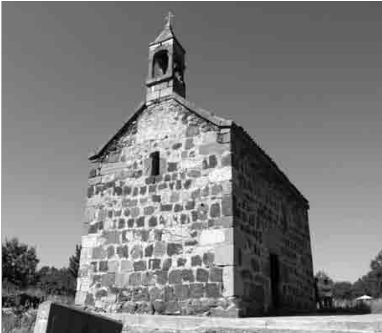
St. Gevorg Church of Mashavera (Gorenjuk) Village from the south-west
