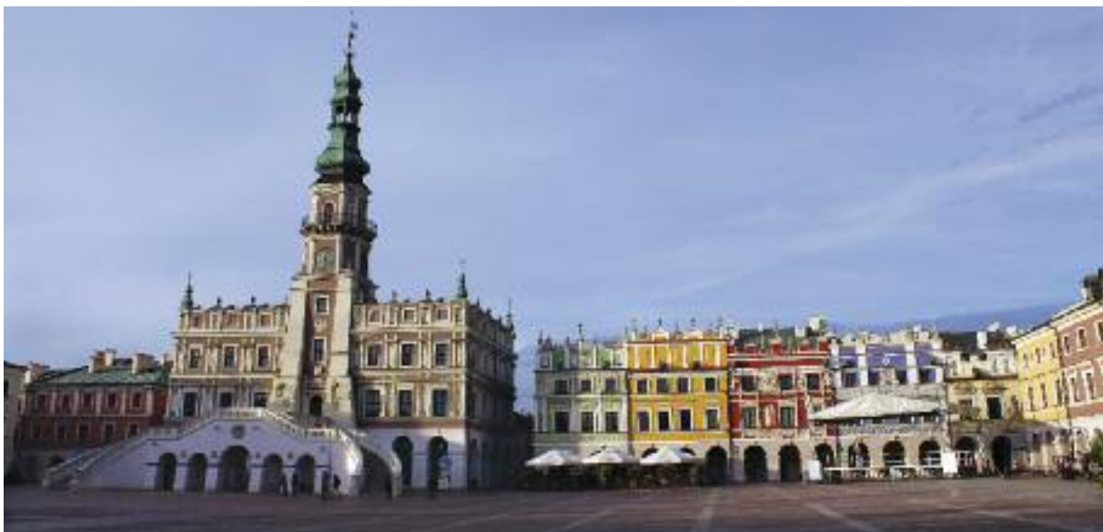
Partial views of the city walls; the Old Lublin and Old Lviv Gates; Rynek Wielki Square in the north of which, Ratusz is located (photos by S. Vardanian, 2014)
