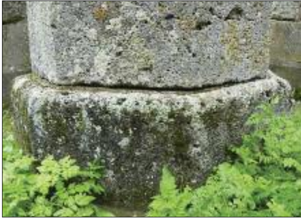
The slit between the north-western facets of the blocks of the pillar base, 2014
