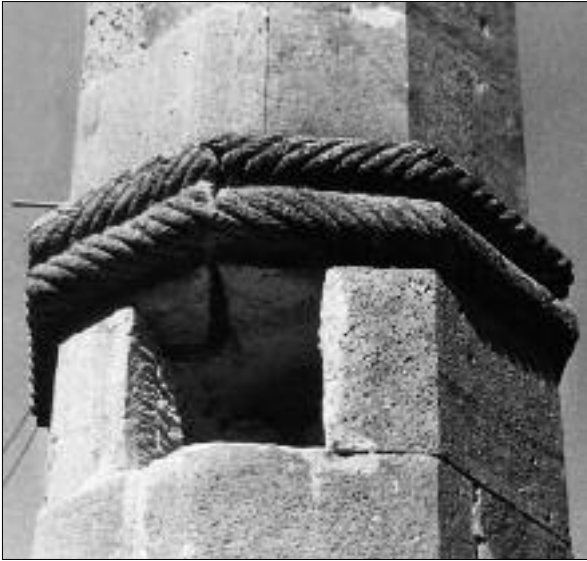
After the displaced stone was taken away, the small opening in the centre of the dividing band became visible, 1987
