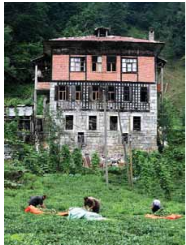
585-587. A mountain village and houses in Hamshen 588. A partial view of Kayakend Village, Hamshen 589. A mountain village in Hamshen
